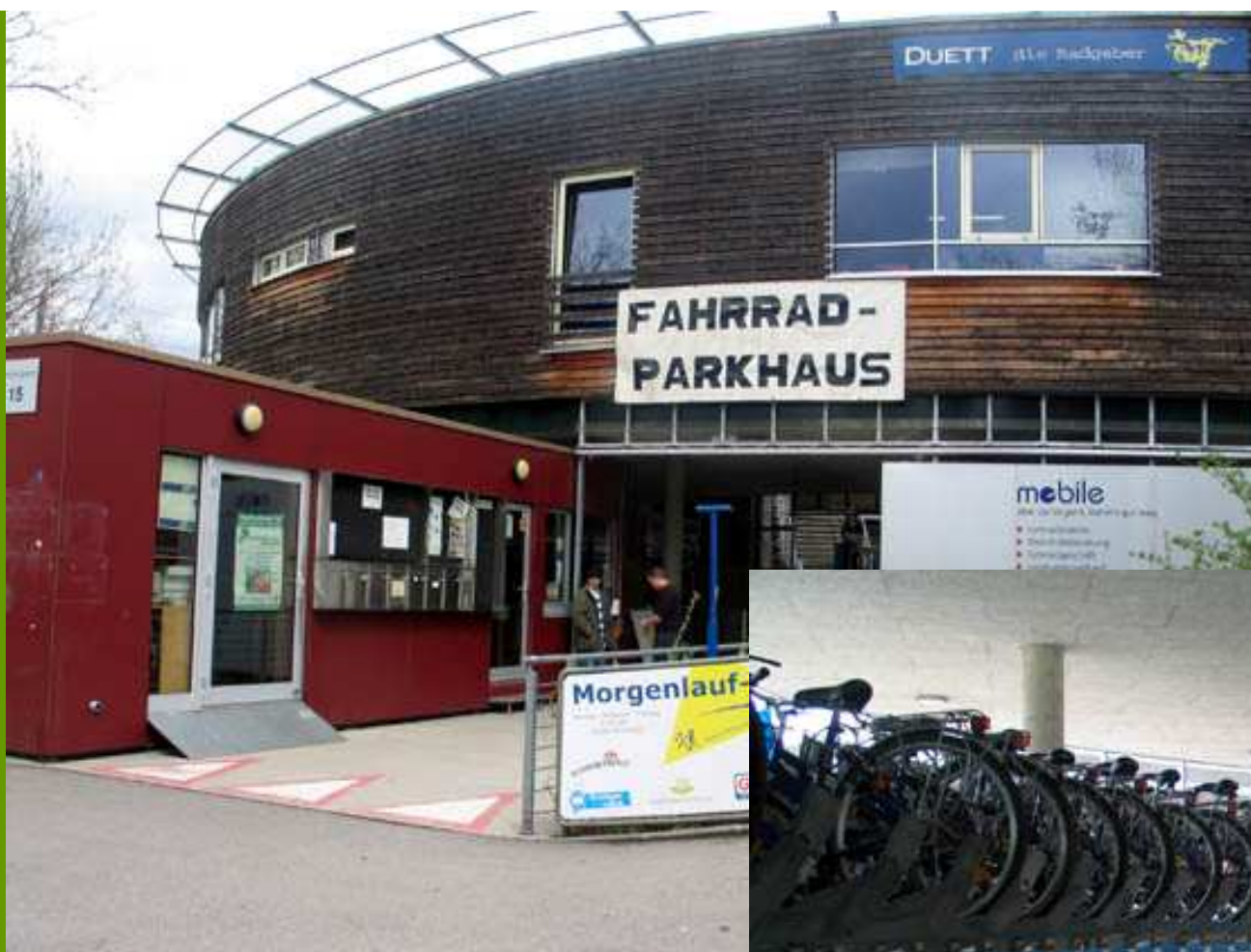
Fahrradparkhaus in Freiburg
